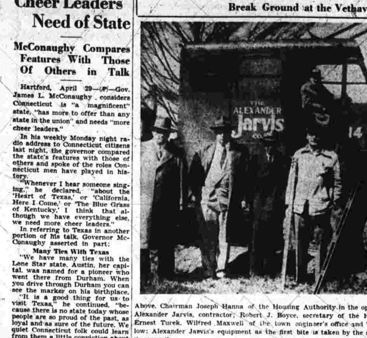
Above: Chairman Joseph Mann of the Housing Authority in the operator's seat; standing left to right: Alexander Jurek, contractor; Robert J. Boyce, secretary of the Housing Authority; Frank Steele, Ernest Turck, Wilfred Maxwell of the town engineer's office and Town Engineer James Sheehey. Below: Alexander Jarvis's equipment as the first bite is taken by the shovel after bulldozer has rolled back to the topsoil.
